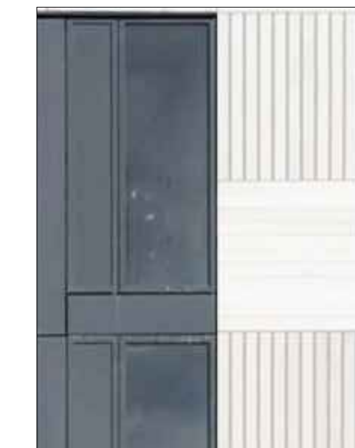
2. DARK COLOURED SPANDREL PANELS
